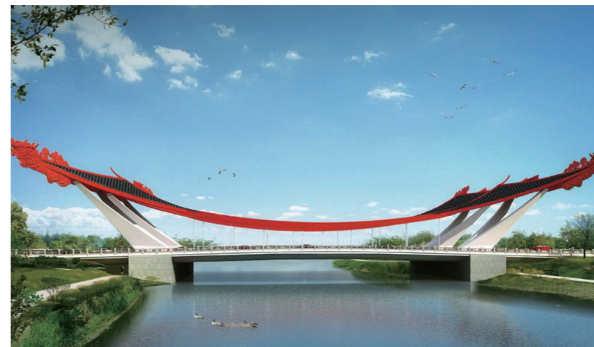
Yulong Yuxi Bridge (2000 tons)
