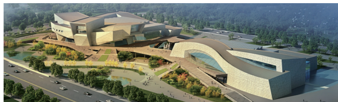
Qufu Olympic Sports Center (4500 tons)
